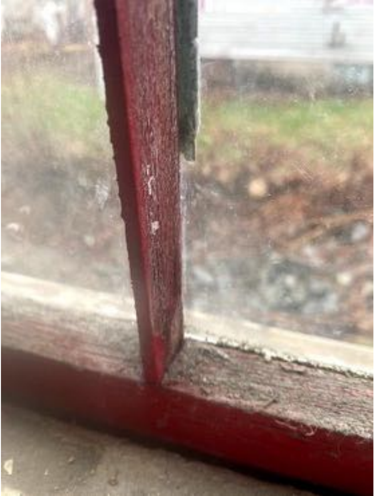
The slight concave curve of the muntins is typical for sash built from 1830-1850.
